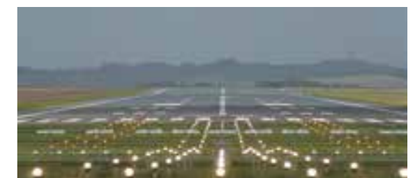
Runway at King Shaka International Airport Durban, South Africa
